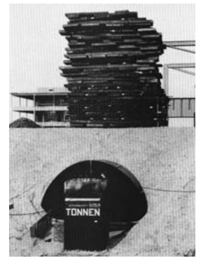
1962 Large-scale load carrying test (> 1000 tons)
