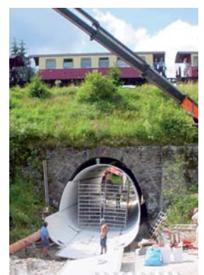
2004 Rebuilding of tunnel with MultiPlate
